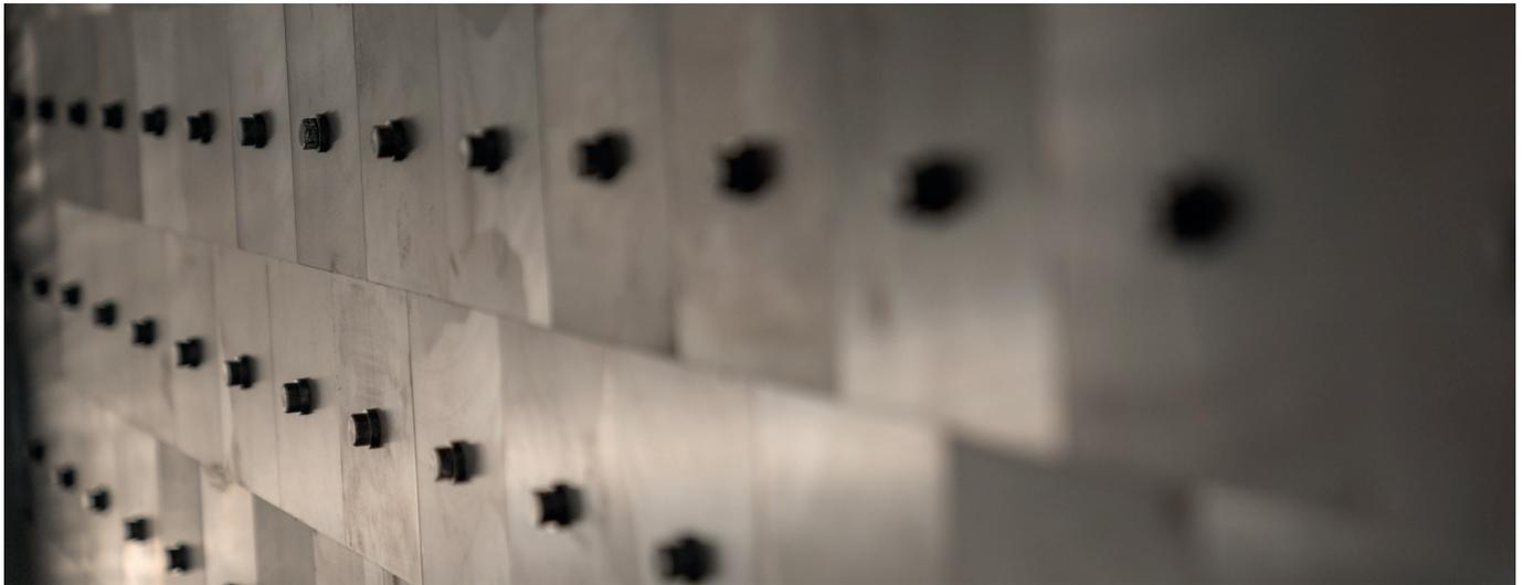
Our 3610 series Ferrite absorber tile is the industry standard solution and exhibits excellent overall performance versus cost. It is an attractive alternative to traditional, large, foam-type absorber materials for new anechoic chambers or for upgrading existing rooms for radiated emission and immunity measurements.
