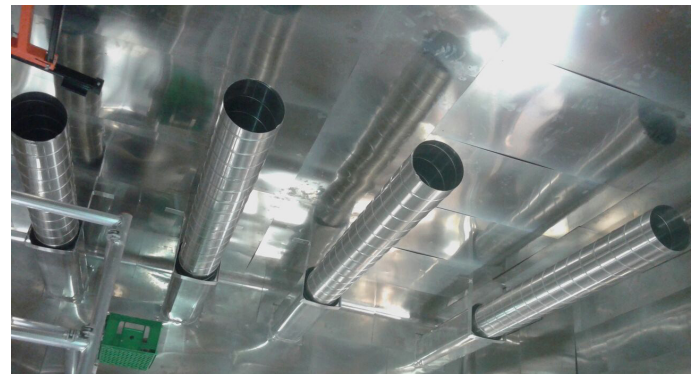
Magnetically shielded Faraday cage with ventilation cylinders, during construction
