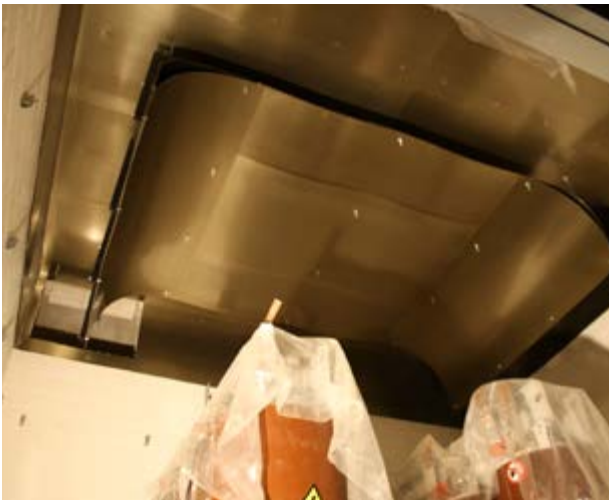
Customer-specific ceiling shielding with MuFerro
