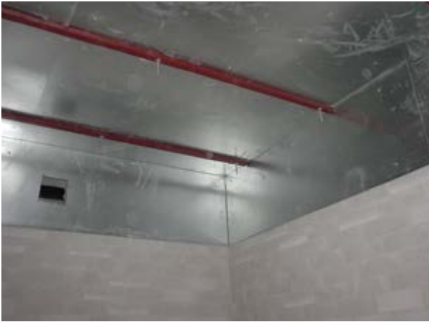
MuFerro 6800 metal shielding structure transformer room
