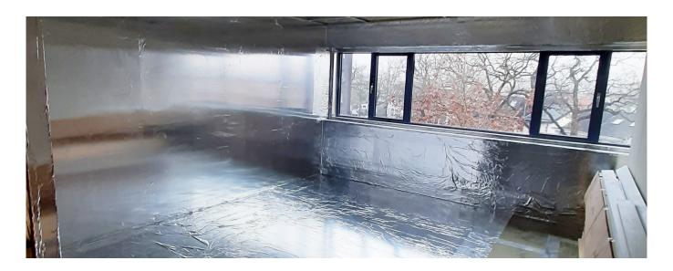
Amucor foil has high attenuation properties in the electrical field (up to 110 dB) as well as in the magnetic field (see shielding performance table).
